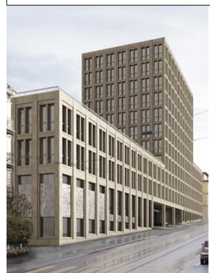
LEE building, Leonhardstr. 21
